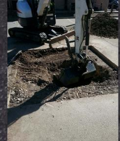
Full depth repair is the digging out of the existing asphalt, to the stone (sometimes more) and putting back new stone, base asphalt and surface course asphalt in lifts. Each lift is compacted before the new one is installed. Once the repaired area is flush with the original or exisitng pavement, edge sealing will smooth transitions and prevent moisture penetration.
