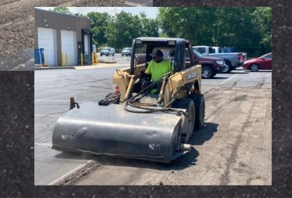
Mill patching is typically done when a client does not want to have any transitions that are inconsistent with the rest of the pavement. Because a mill patch is flush with the exisiting asphalt, the transition from new to old is nearly seamless in nature.
