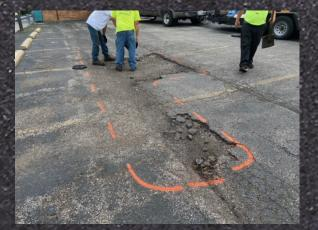
A Surface Patch is cleaned and then tacked for adhesion, with an SS-1 Emulsion tack. Then asphalt is placed in the hole and the surrounding areas, and then compacted to maximum density to form the patch or repair. Edge sealing can then be done to ease
